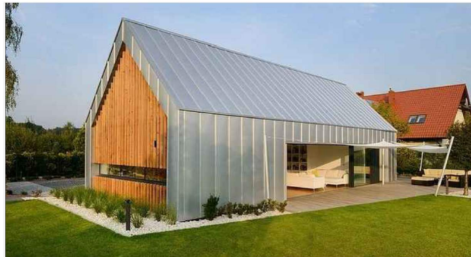
Dwellings to pick up on barn conversion language with metal cladding to elevations and roof.
