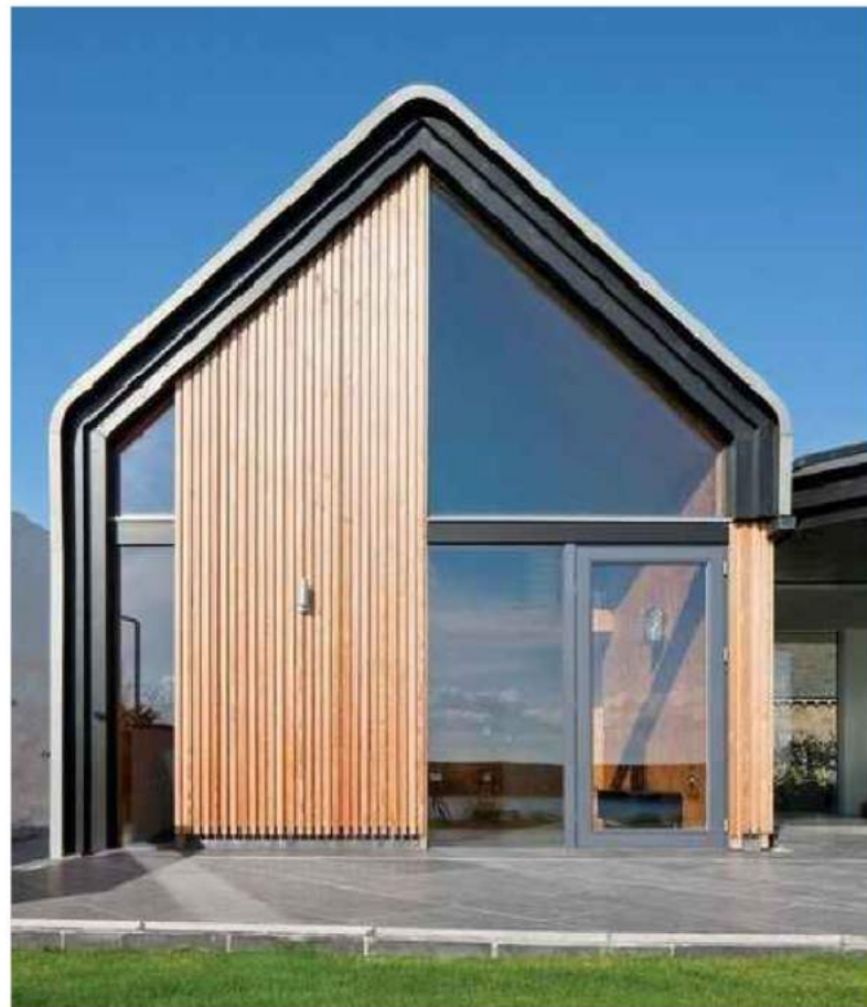
Single storey with double height glazing
